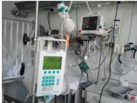
Fig.5.2: Hospital electrical equipment
